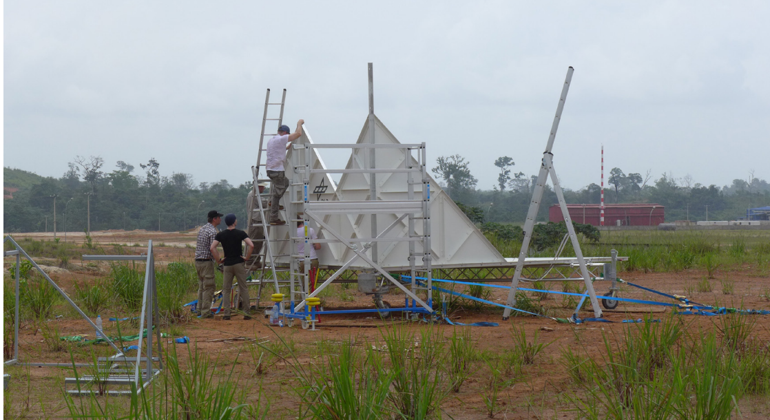
Image front page: © Linder; The assembled 5 meter reflector in the workshop Image right: © Linder; The reflector during the assembly in Garbon
